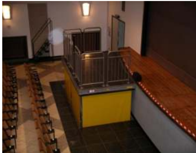
loading lift platform for material transport up to a stage with gap protection and socket railing
